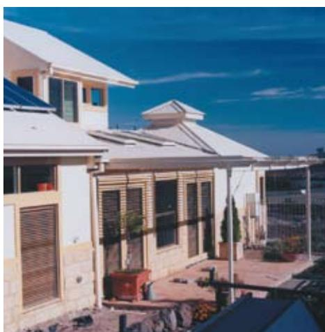
The west windows are designed as 'zen' picture windows to frame the view, limiting the thermal load and solar penetration.
