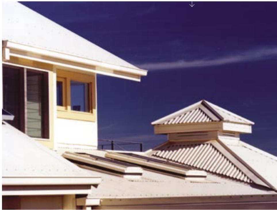
sustainability and renewable energy. The gas-boosted solar hot water system has been installed on the north-facing roof above the kitchen in order to be close to the bathroom, the most frequent draw-off point to avoid heat loss from long lengths of piping. Beside it is the grid-connected photovoltaic array, which generates about one quarter of required household electricity.
